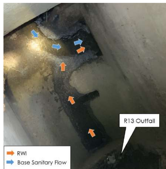
Figure 8-4. R13 Regulator Structure Photo, Facing Down; September 2020
