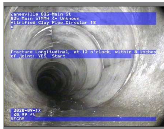
Photo: Unknown_825 Main STMMH_20200917_1314_FL_17092020131418.JPG, 00:02:43 40.91FT, Fracture Longitudinal, at 12 o'clock, within 8 inches of joint: YES, Start
