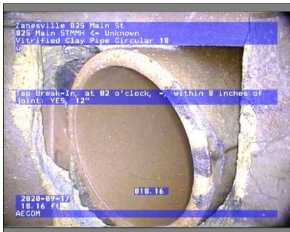
Photo: Unknown_825 Main STMMH_20200917_1312_TB_17092020131216.JPG, 00:00:53 18.16FT, Tap Break-In, at 02 o'clock, -, within 8 inches of joint: YES, 12"
