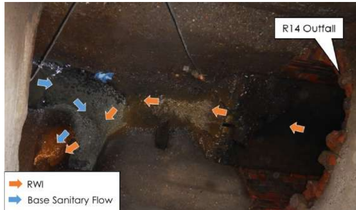
Figure 8-5. R14 Regulator Structure Photo, Facing Down; September 2020
