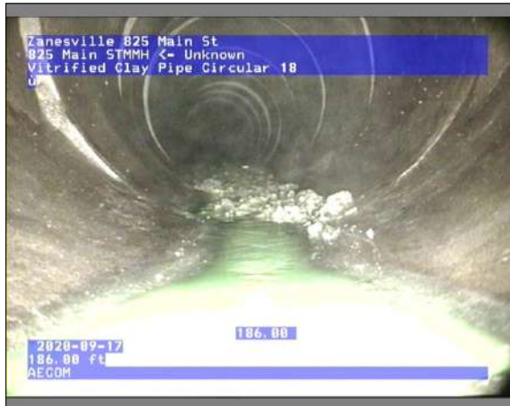
Photo: Unknown_825 Main STMMH_20200917_1353_MSA_17092020135317.JPG, 00:20:44 186FT, Survey Abandoned / Could not advance
