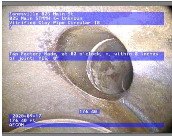
Photo: Unknown_825 Main STMMH_20200917_1323_TF_17092020132349.JPG, 00:09:46 176.4FT, Tap Factory Made, at 02 o'clock, -, within 8 inches of joint: YES, 8"
