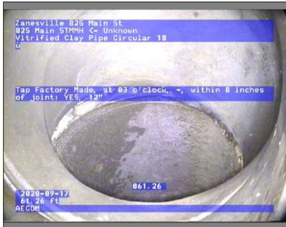
Photo: Unknown_825 Main STMMH_20200917_1315_TF_17092020131508.JPG, 00:03:18 61.26FT, Tap Factory Made, at 03 o'clock, -, within 8 inches of joint: YES, 12"
