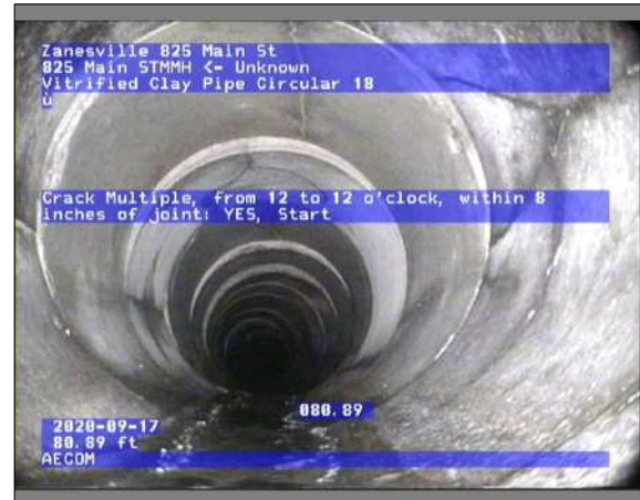
Photo: Unknown_825 Main STMMH_20200917_1316_CM_17092020131605.JPG, 00:04:03 80.89FT, Crack Multiple, from 12 to 12 o'clock, within 8 inches of joint: YES, Start
