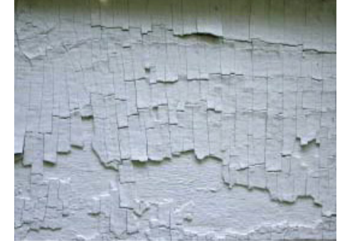
Alligatoring paint on exterior siding.
