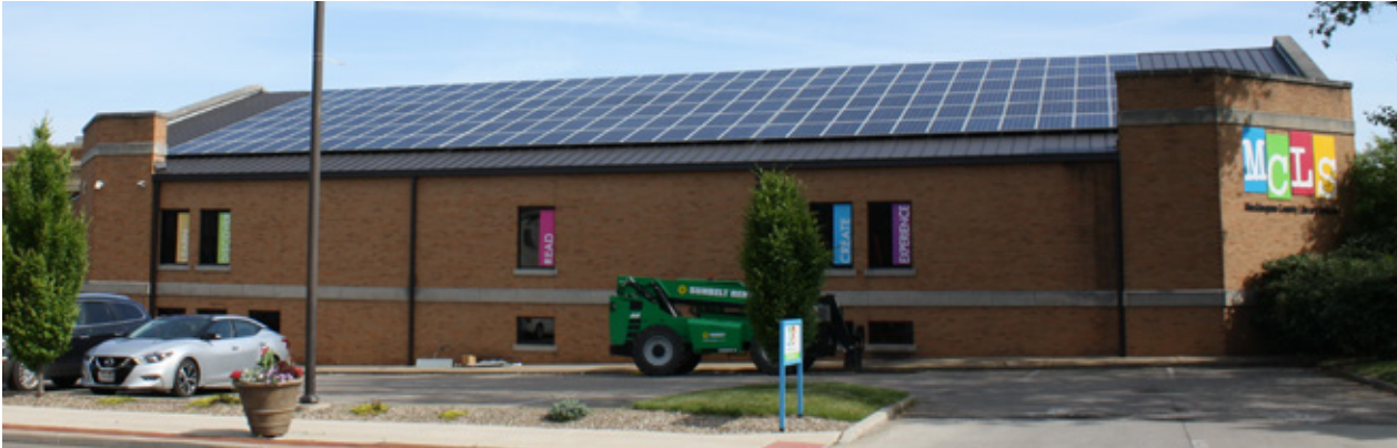
Addition to the Muskingum County Public Library features building integrated solar panels.
