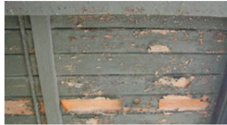
Paint failure on the underside of a wood canopy.
