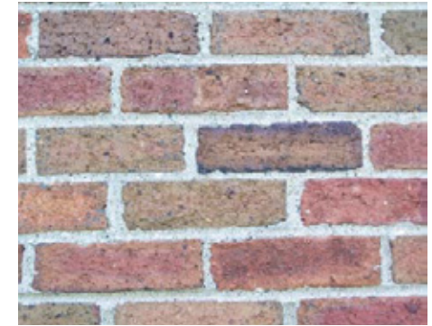
Damage to brick caused by sandblasting.
