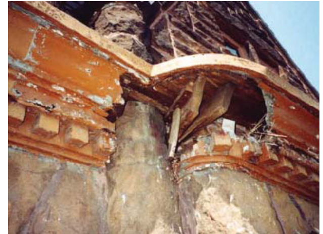
A painted lead-coated copper cornice is missing elements due to advanced deterioration of metal.
