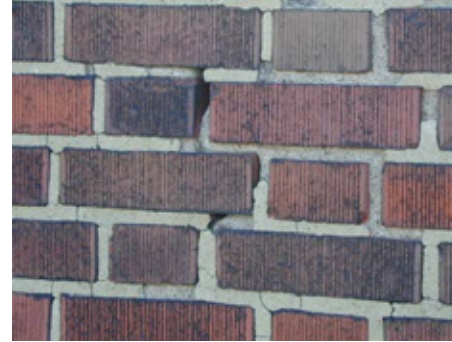
Previous poor repointing. Repointing mortar is falling out of joint due to improper execution.
