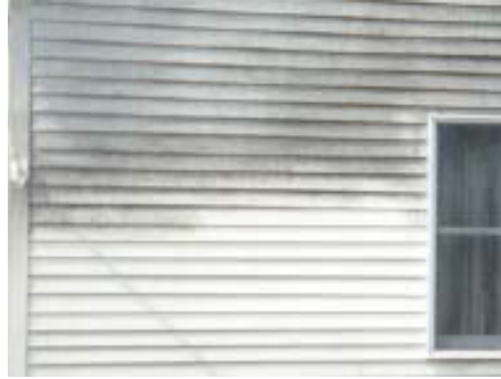
Mildew on painted exterior siding.
